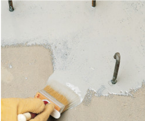
Applying Eporip by brush on construction joint
